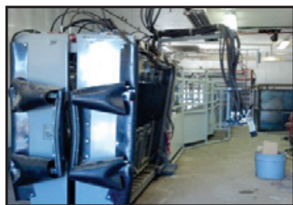
Wulf Cattle Handling facilities on their ranches for processing, treating and breeding cattle consist of a bud box and free flow tub concept.
